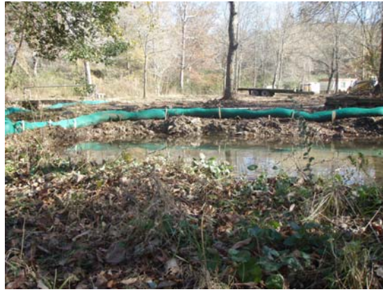
Above Tapawingo Springs, after the removal of home and outbuildings. The blue mulch socks prevent silt from entering the springs. Right The dilapidated home and outbuildings on the Springs, and on demolition day.
